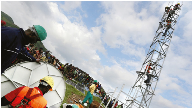
3 It doesn't take long for the tower to take shape.
