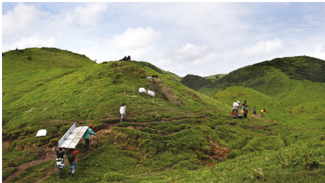
1 Workers bring the equipment to the tower site.
